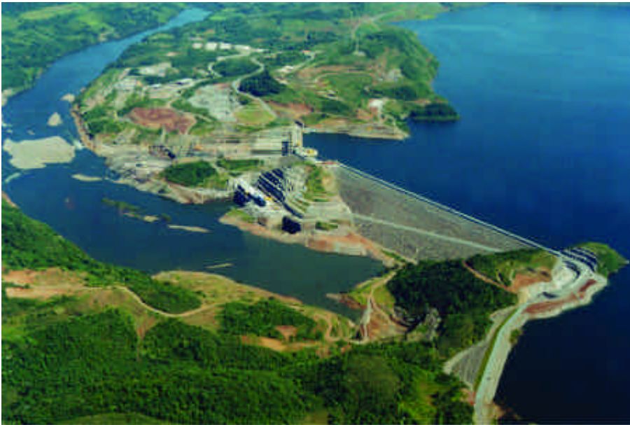
As more countries create competitive markets for electricity in Latin America, hydropower stations such as the newly commissioned 1,140-mw Machadinho in Brazil (shown above) gain in value, owing to the special services they can provide to the grids.
